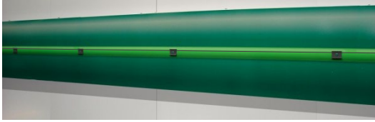
Figure 9: Chalk-line and mounting clips installed
