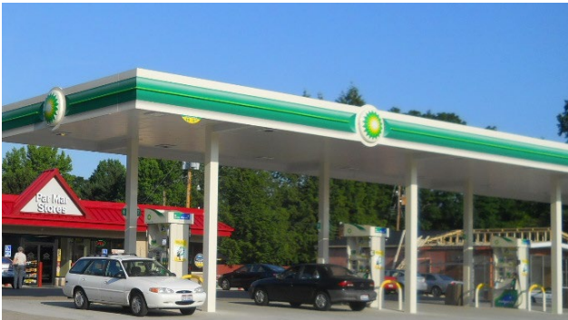
Sides of fascia with Unlit LightBar
