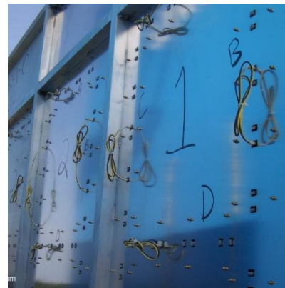
Figure 13: Modular LED digits wiring from behind face
