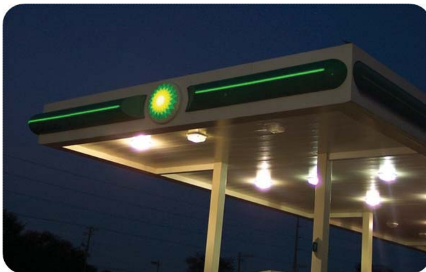
CANOPY BULLNOSE LED & INSTALLATION
